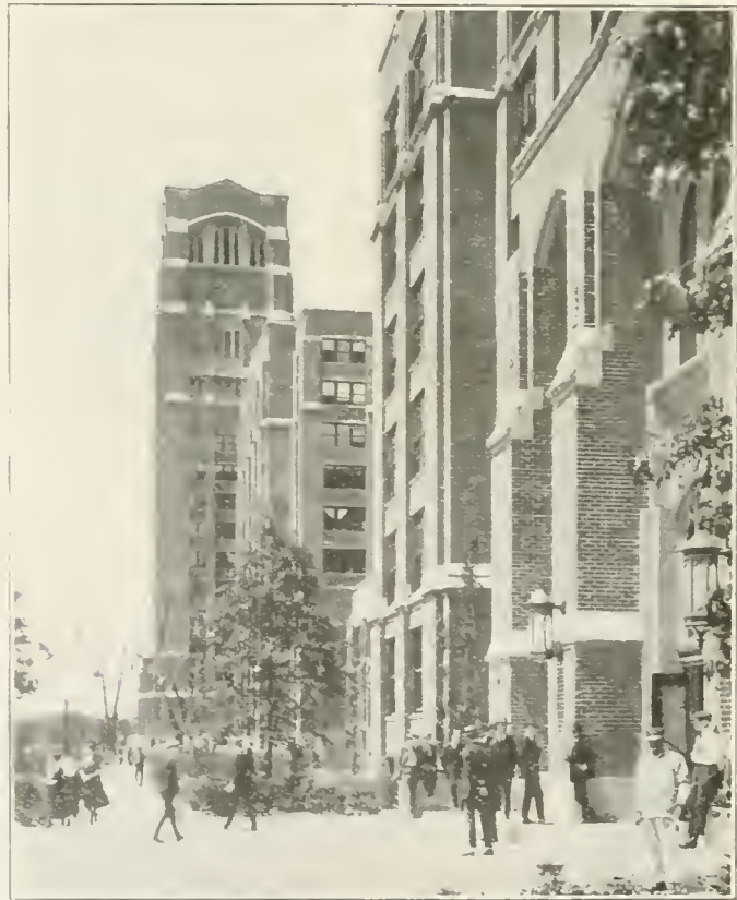
The tower that dominates the group is not for its ornamental effect at all, but to meet the very essential requirement of providing a place for the sprinkler tanks.
